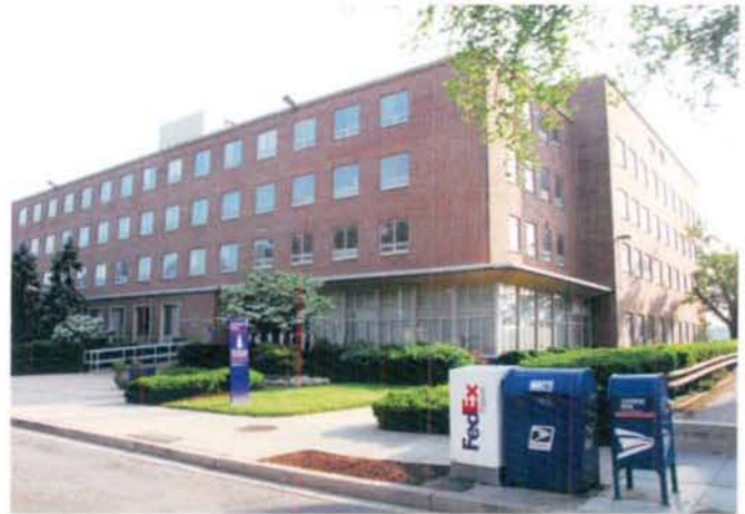
Photo 5-28: View of Johnson Administration Center
