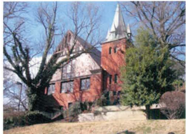
Photo 5-19: View of Rankin Chapel West Elevation
