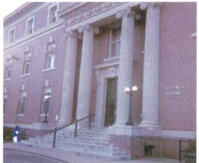
Photo 5-8: View of C.B. Powell Building
