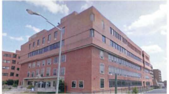
Photo 5-10: View of College of Dentistry Building
