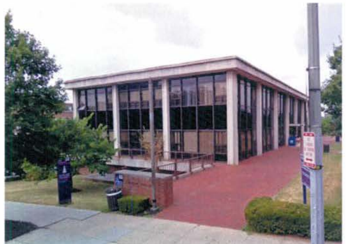
Photo 5-6: View of Inabel Burns Lindsay Hall/School of Social Work
