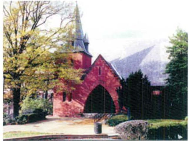
Photo 5-18: View of Rankin Chapel East Elevation
