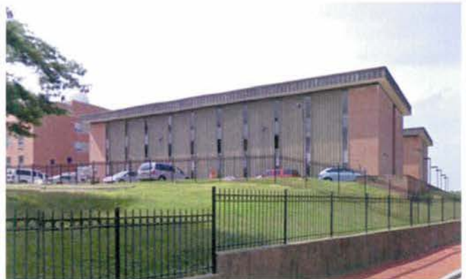
Photo 5-5: View of Academic Support Building School of Education
